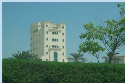
BAHRAIN: TARIQ HOSPITAL 39 units of 1500L calorifiers
