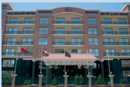
BAHRAIN: TAJ PALACE HOTEL ISSA TOWN 2 units of 1500L calorifiers
